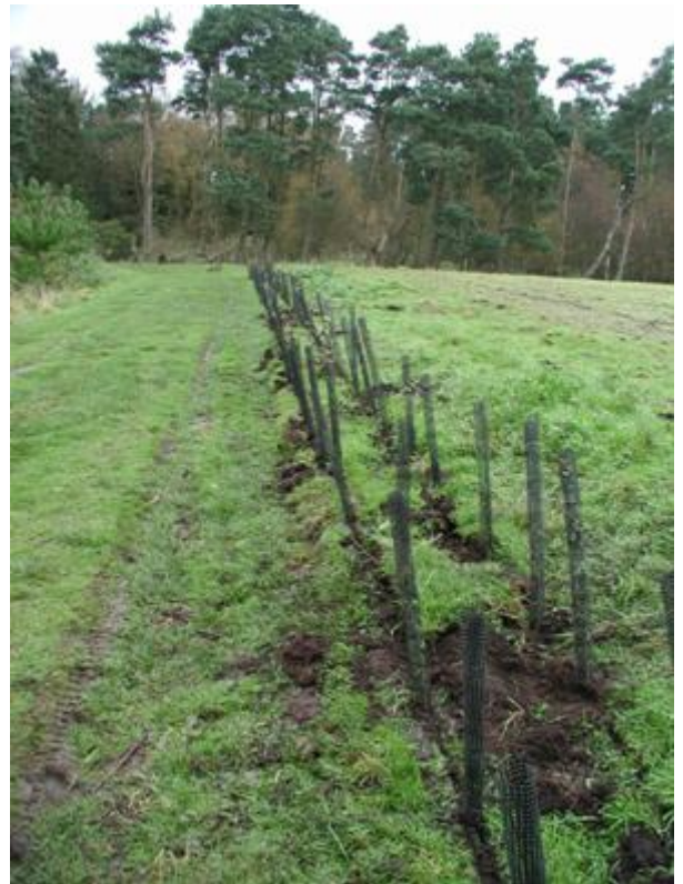
Newly planted hedge in double rows with protective guards
